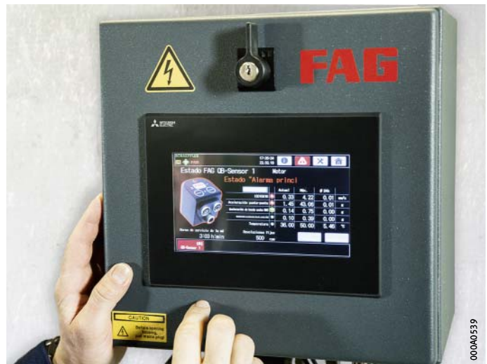
Figure 2 Online monitoring system FAG SmartQB
