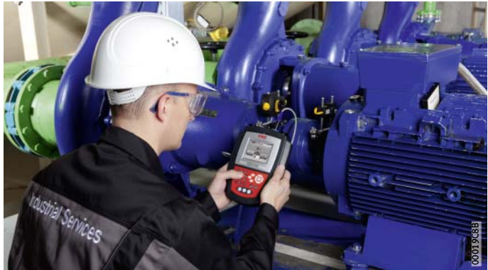
Figure 6 Shaft alignment device FAG Top-Laser EQUILIGN
