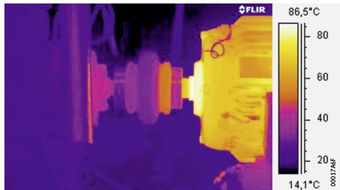
Figure 5 Thermography® FLIR systems Approval inspection of new plant
